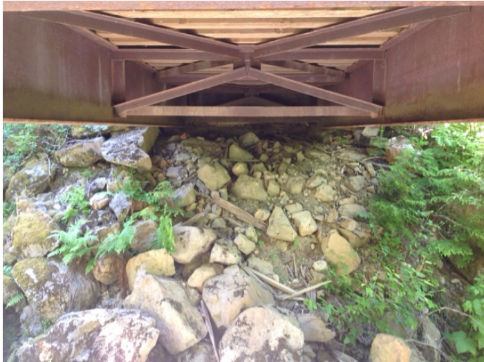
Left Bank Abutment when facing downstream
