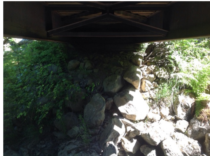
Right Bank Abutment when facing downstream
